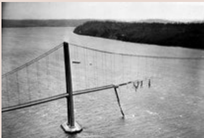
Collapse of the Tacoma Narrows Bridge
