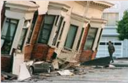
Collapsed apartment building in San Francisco, October 18, 1989, the day after the massive Loma Prieta earthquake
