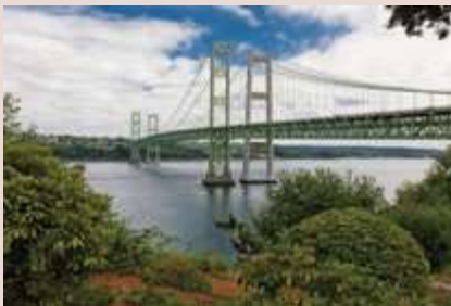
The rebuilt Tacoma Narrows bridge (1950) and new parallel bridge (2009)
